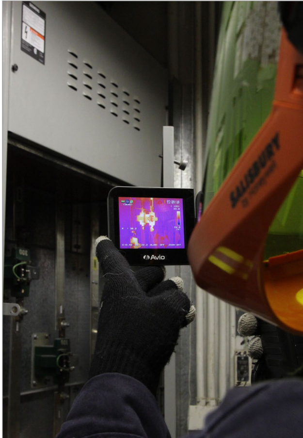
Figure 14. Infrared thermal scan. Source: Heartland Farm Mutual, Waterloo, Ontario.
