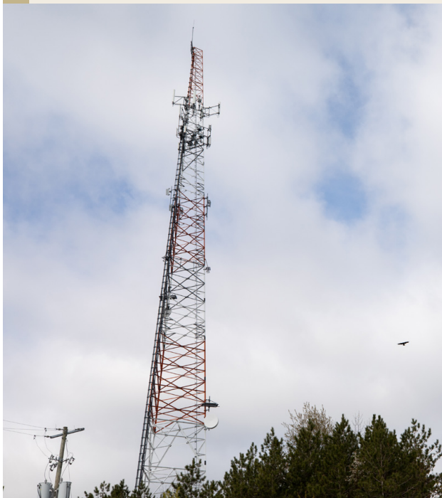
A cell tower in Ontario.
