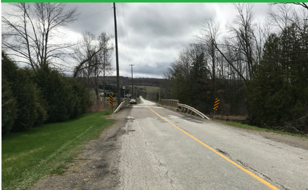
Grange Sideroad bridge before rehabilitation in Caledon.
