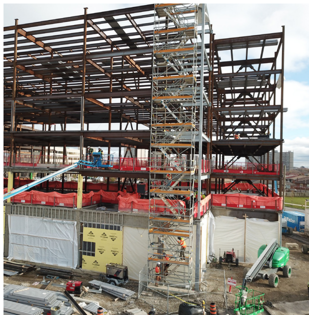
Construction at Humber River Hospital (long-term care accelerated build) in Toronto.
