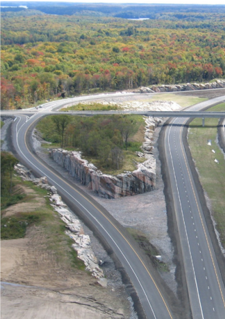
Highway 400 rehabilitation at Highway 141 between Parry Sound and Muskoka Lakes.
