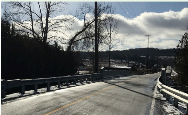
Grange Sideroad bridge after rehabilitation in Caledon.
