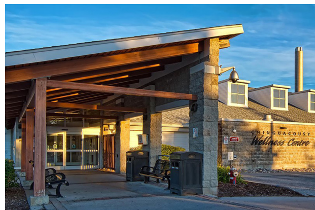
Rehabilitation of the Chinguacousy Wellness Centre in Brampton.
