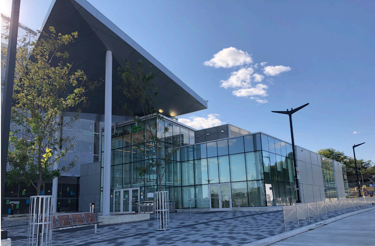
The new Cooksville GO station in Mississauga.
