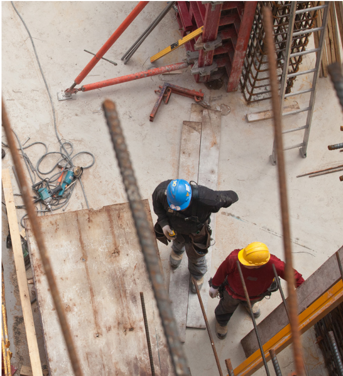
Construction workers at SickKids Research and Learning Tower in Toronto.
