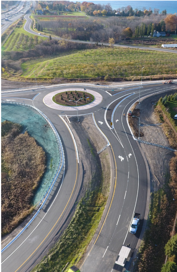
Highway roundabout in Southern Ontario.
