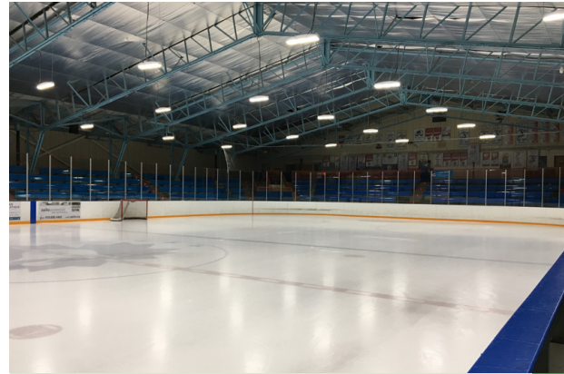
Upgrading the George Bell Arena in Toronto.
