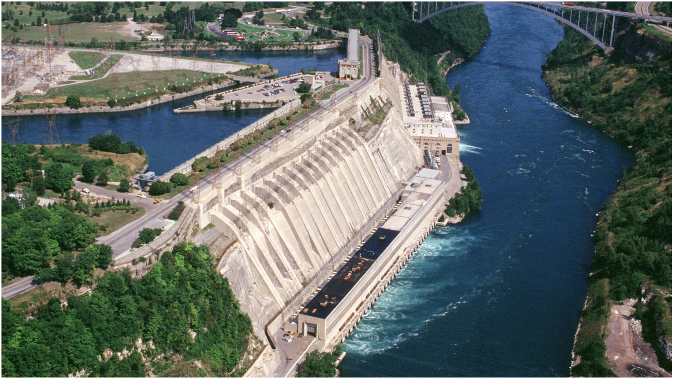
Sir Adam Beck Hydroelectric Generating Station.
