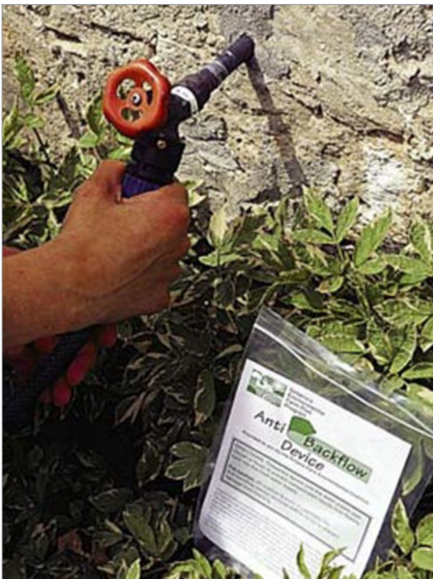
Figure 3. Install anti-backflow devices on all outdoor faucets. The devices cost only a few dollars and are available in brass or plastic.
