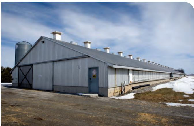
Figure 26. Exterior of a turkey barn.
