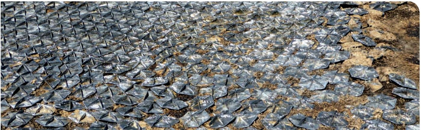
Figure 40. Round liquid manure storage with floating permanent cover comprised of plastic hexagon discs (L2).
