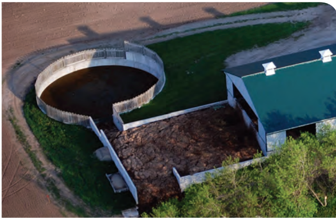
Figure 38. Uncovered liquid runoff storage (L1).
