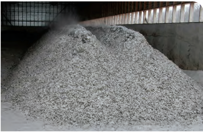
Figure 31. Covered solid manure storage (V2) with slatted walls.
