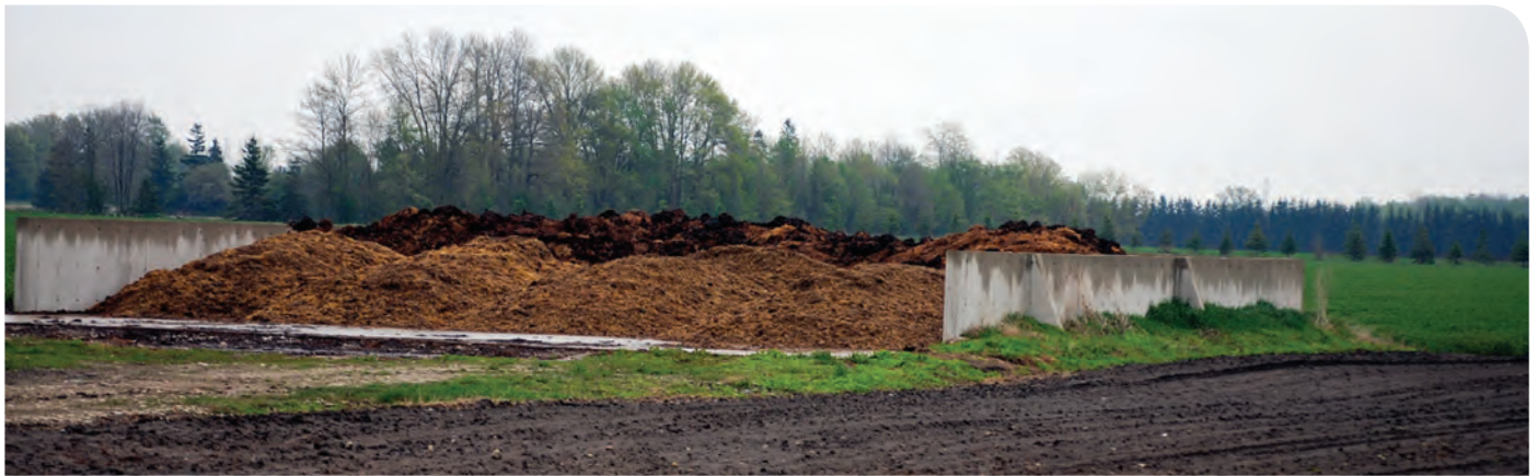
Figure 33. An outdoor, uncovered solid manure storage (V3).
