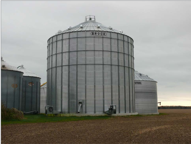
Figure 1. A large storage bin with two centrifugal fans mounted through the sidewall. This bin has numerous vents around the roof. The vents are placed about 2 m (6 ft) back from the eave of the roof.
