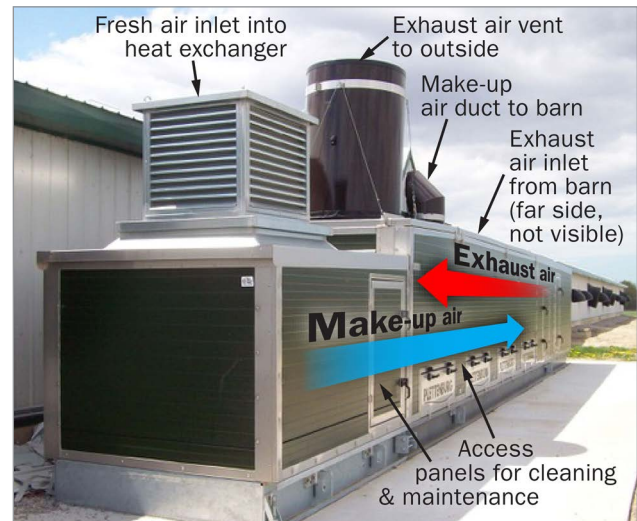
Figure 3. This heat exchanger is designed to handle 100% of the ventilation in winter months. The core is located inside the large cabinet. Exhaust air and make-up air travel in opposite directions through the core, and heat moves between them.
