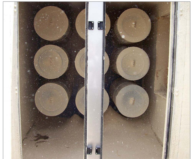
Figure 5. This heat exchanger uses cylindrical air filters, with an automatic back-flush feature to clean them at regular intervals. The filters are easily accessible for removal and cleaning.
