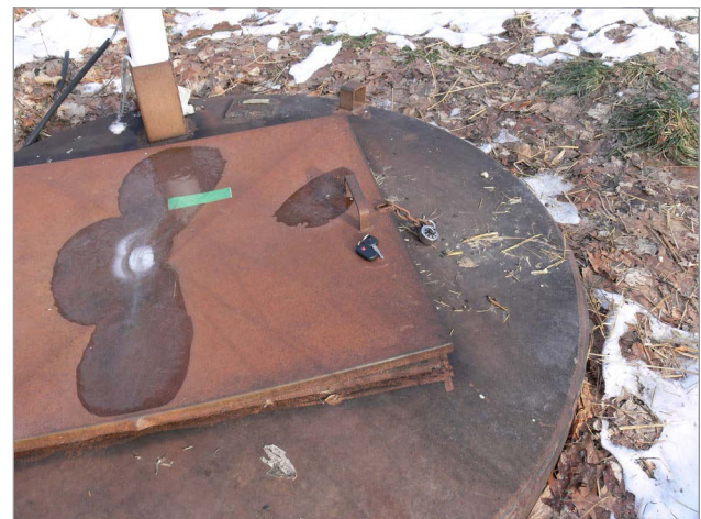
Figure 6. Hatches must be large, strong, easy to open during any kind of weather and locked between uses. Note the air vent beside the hatch, which is about 10 cm x 10 cm (4 in. x 4 in.), large enough to encourage flies and beetles that scavenge on deadstock to find their way into the vessel.
