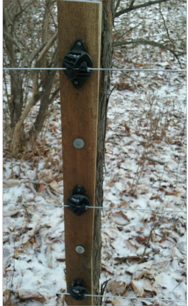
Figure 3. For “living fenceposts,” electric fencing insulators should first be affixed to mounting strips that can be loosened off the growing trees by backing-off screws. Source: Brett Chedzoy.
