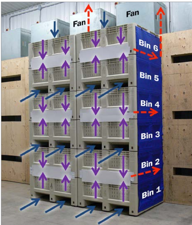
Figure 4. Serpentine horizontal/vertical airflow system example (photo by Hugh Fraser, OMAFA).
