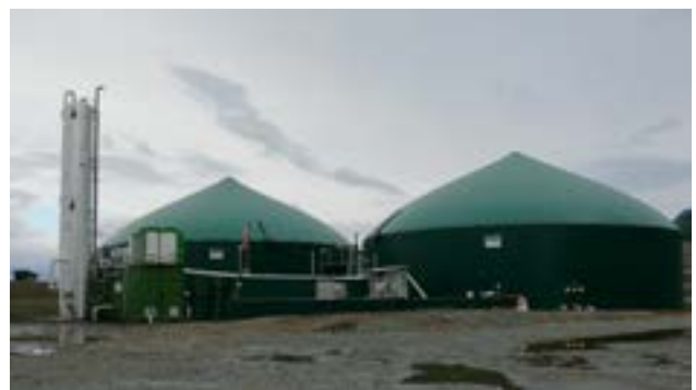
Figure 1. A farm-based biogas system producing renewable natural gas in British Columbia. The upgrader system that concentrates the methane gas to meet natural gas standards is located on the left side of picture.
