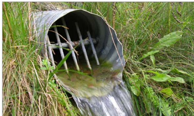
Figure 3. Outfall pipe with rodent guard installed.
