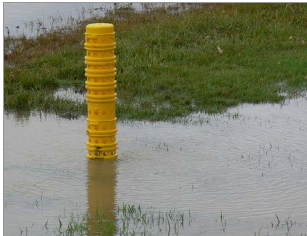
Figure 9. Surface water inlet.
