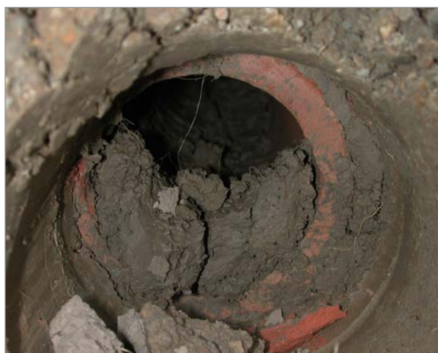
Figure 7. Drain pipe containing a significant amount of sediment caused by a blowout.
