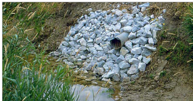
Figure 4. Outfall pipe with erosion control located above the water level.
