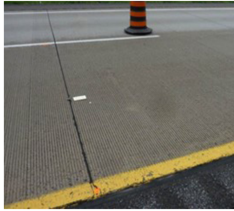
Figure 7a: Concrete joint deterioration without surface signs.
