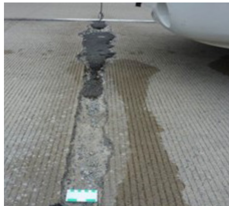
Figure 6a: Concrete with underlying joint distress visible from the surface.
