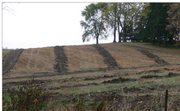
Figure 3. Recently installed subsurface drainage system left to settle naturally.
