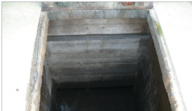
Figure 3. Pump-outs with baffles will cause the head spaces in unvented storages to become pressurized once the manure level rises above the bottom of the baffle.
