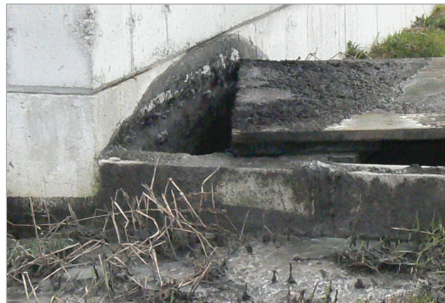
Figure 4. A manure pit cover that was pushed off by manure foam.
