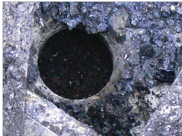
Figure 2. This open pull plug hole is the suspected source of methane from the lower pit that resulted in a nursery barn fire.
