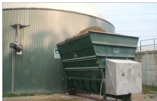
Figure 3. Hopper holding corn silage to be fed into digester.
