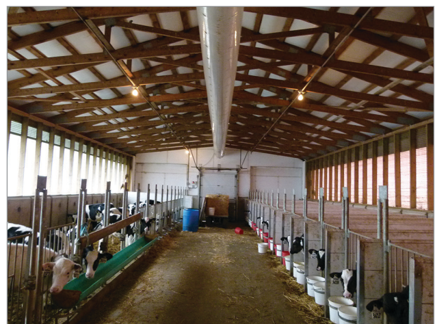
Figure 1. PPAT systems improve calf barn ventilation.
