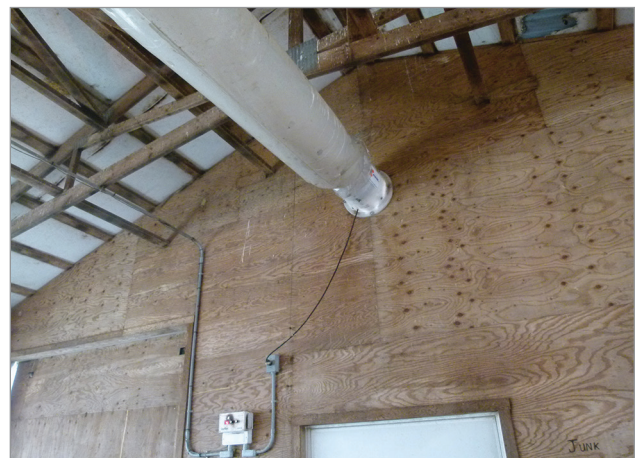
Figure 2. The air tube is sized to match the fan capacity.
