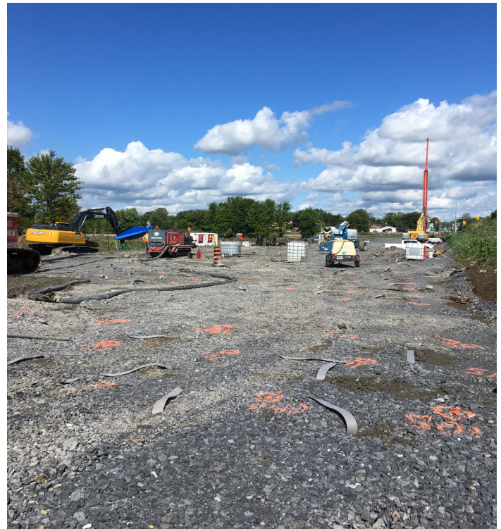
RI installation at the south embankment. The orange markings indicate the surveyed locations for RIs and wick drains.
