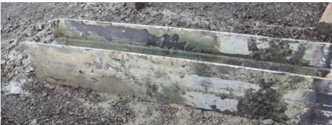
Figure 5: The piles at the Highway 401 and Hallecks Road interchange show minimal corrosion.
