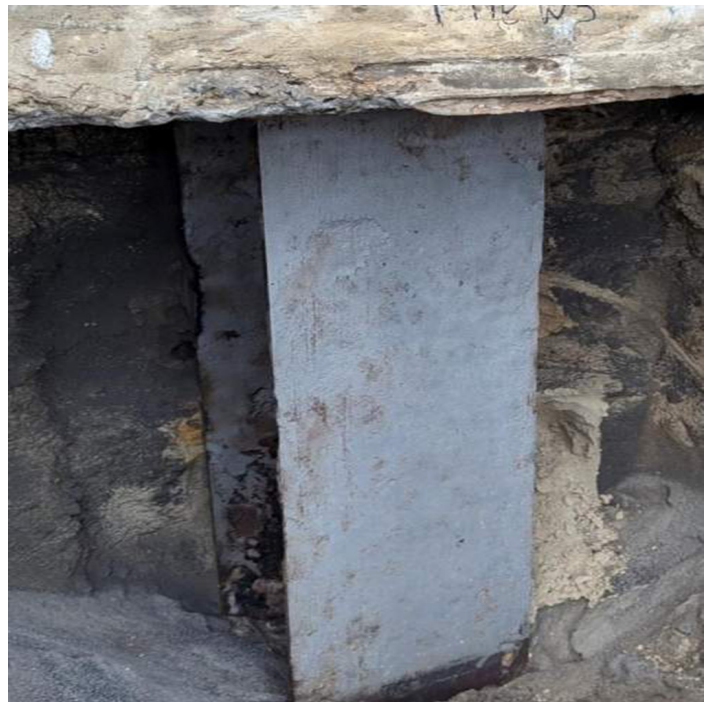
Figure 4: Post-blast cleaning of pile W3 at Woodroffe Avenue.
