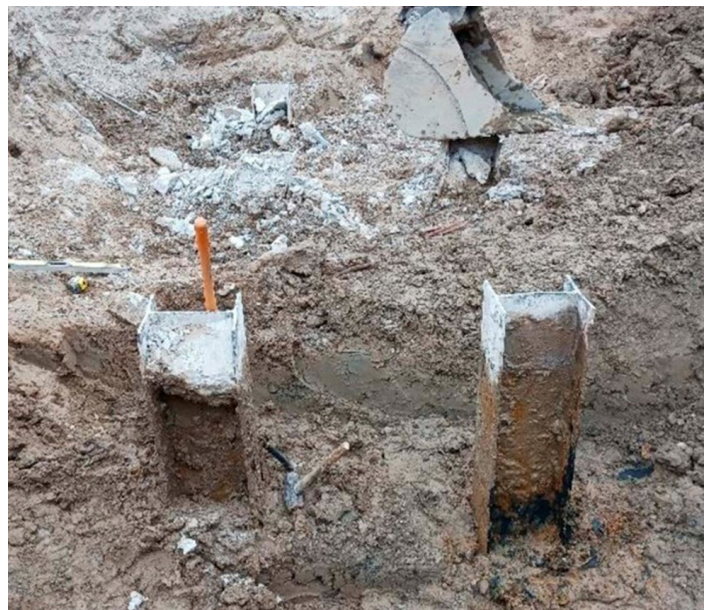
Figure 2: Exposed H-piles at the Leslie Street interchange.
