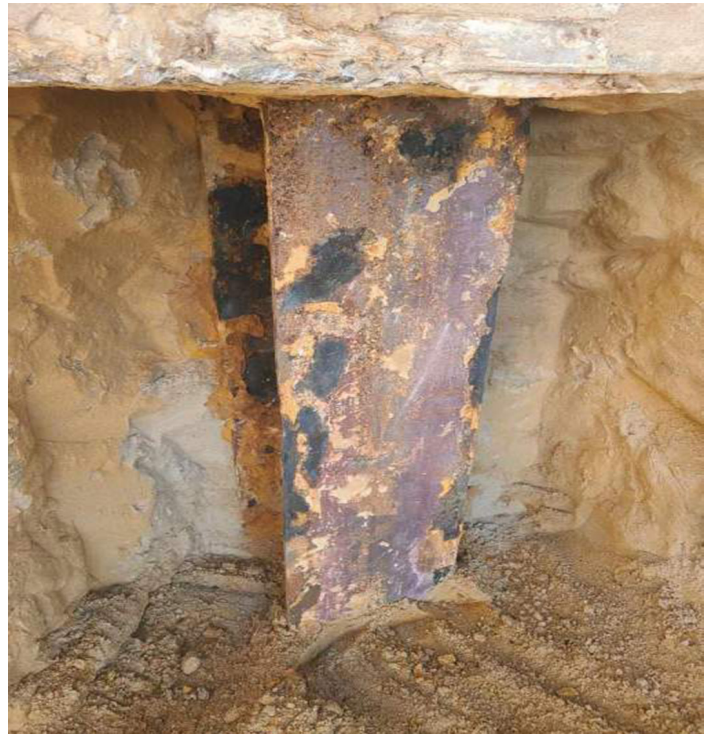
Figure 3: Pre-blast cleaning of pile W3 at Woodroffe Avenue.
