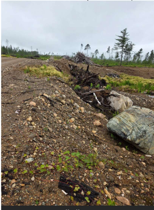
Figure 10, Aggregate pit close to road with steep ditch line
