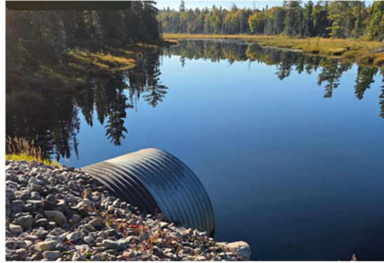
Figure 5. A well installed culvert.
