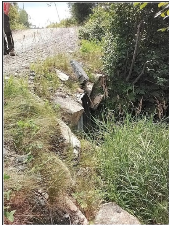
Figure 8: Junior-1 Culvert Crossing
