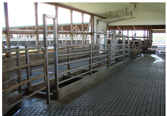
Figure 3. Diamond grooving for improving traction.
