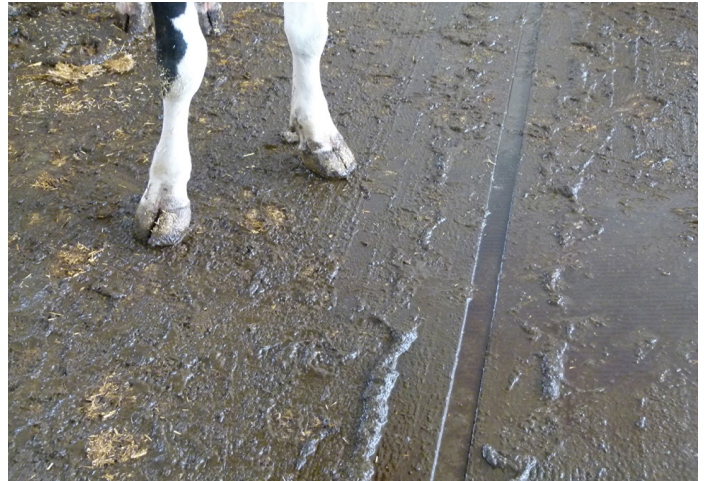
Figure 4. Surface milling improves traction.
