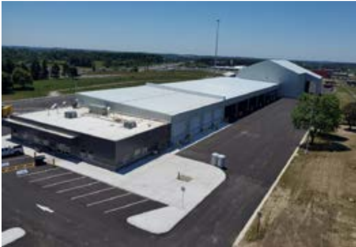
Figure 7: Aerial image of the Ayr MPY during the final stages of construction.
