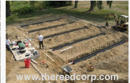
Septic System Upgrades
